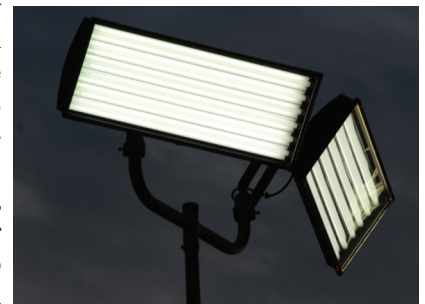
Fluorescent fixtures are new to the outdoor market but use a proven technology.
